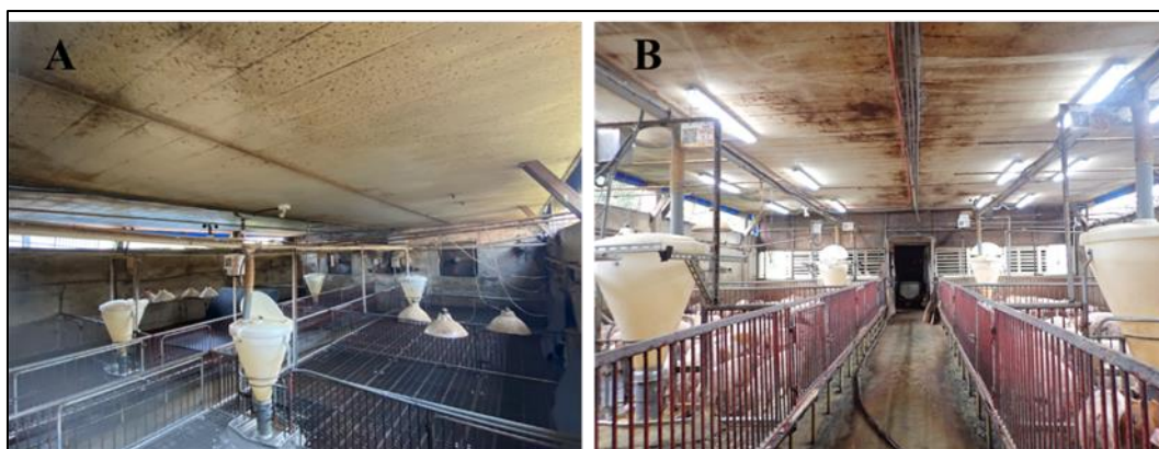
Figure 1 Application of the new-generation LED environmental remediation system in a traditional nursery pig farm. (A) Facility before LED installation. (B) Facility after LED installation.
