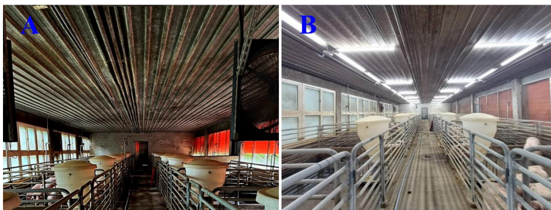
Figure 1 Application of LED-based degradation technology for harmful substances during the growing to finishing stages in an enclosed water-curtain-type SPF pig farm. (A) Before the new-generation LED installation. (B) After the new-generation LED installation
